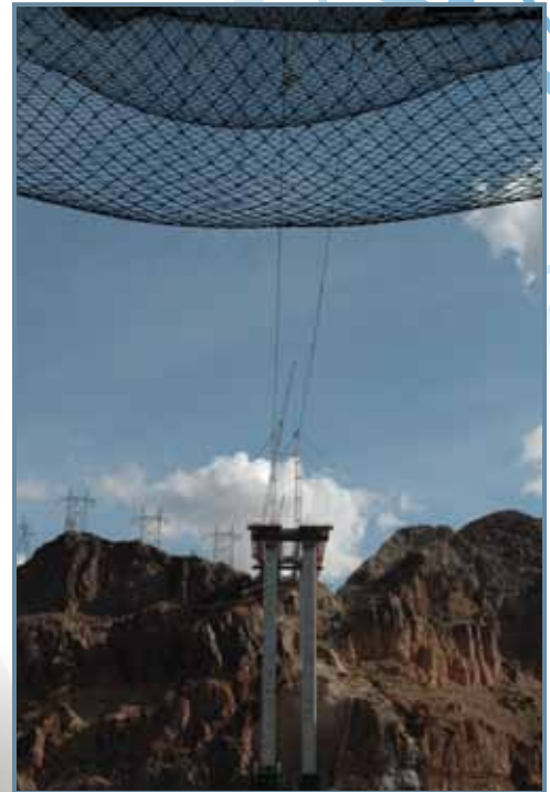
Hoover Dam Bypass Project US 93
