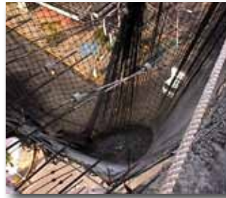
12 cubic feet of concrete caught by safety netting with debris liner.
