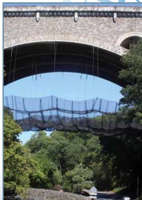
Henry Avenue Bridge, Philadelphia, PA RocBloc Installation by FallProof
